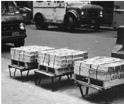
There is no solution to the current crisis without turning away from a fixation on money, (above: gold ingots) toward the concept of economic growth based on high-technology production, demonstrated (at right) by this automated robot spot-welding in a Chicago auto assembly plant.
