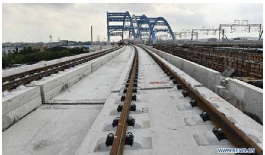
Photo taken on July 31, 2015 shows the last 500 meters of ballastless track of Foshan-Zhaoqing intercity rail line, in south China's Guangdong Province.
