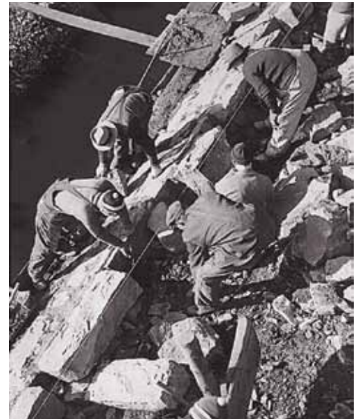
Works Progress Administration (WPA) construction.
