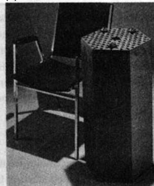
The fuel rods are inserted into holes that are drilled into the hexagonal graphite fuel element blocks, which are 14 inches in diameter and 31 inches long.
