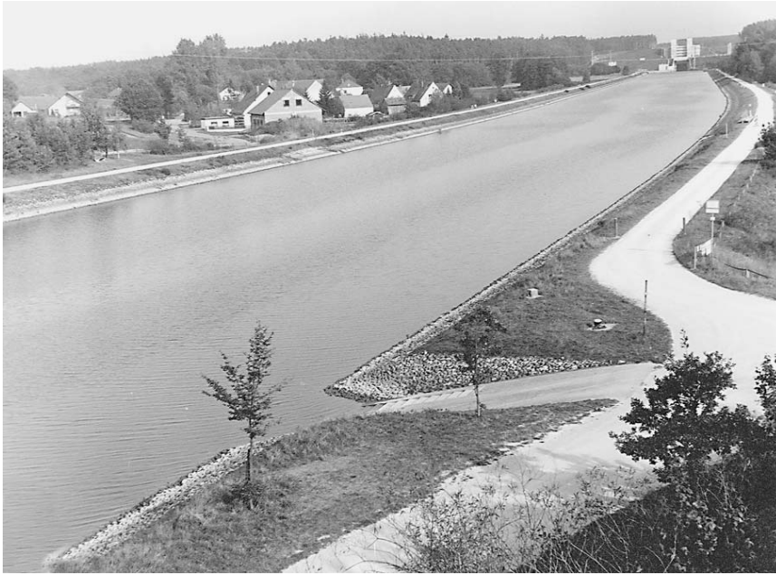
The Main-Danube Canal in Germany, with one of the locks shown in the background. A priority for Balkan reconstruction is that the Danube River be cleared immediately of debris from the war in Yugoslavia, for not only normal but expanded barge traffic. The Balkans cannot become economically and politically stable “without developing commerce around the Rhine-Main-Danube artery from the North Sea to the Black Sea, and without developing a high density of transportation and power conduits, south from the Danube to the Mediterranean and Black Sea.”
