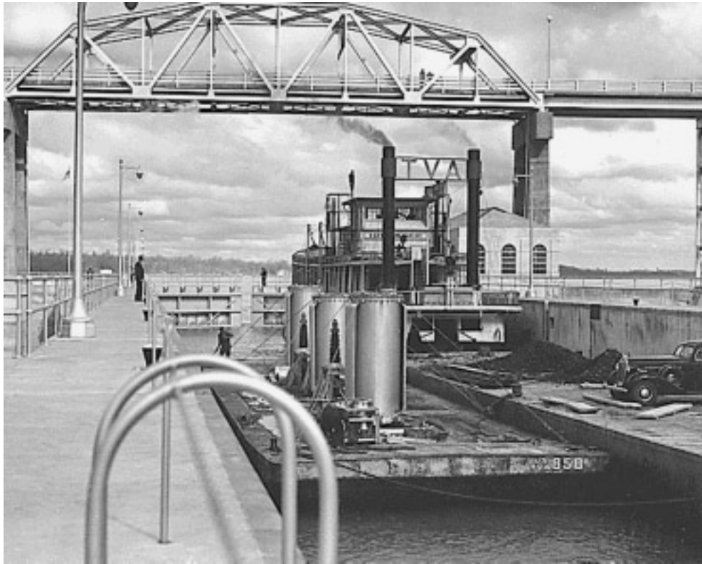
The Tennessee Valley Authority (TVA), the greatest project of the Roosevelt era, transformed that whole section of the southern United States. Here, the Wheeler Dam Navigation Lock in 1942.
