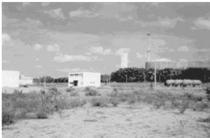
Nuclear plants which desalinate seawater are already in use in several countries; this unit is under construction at the Kalpakkam Nuclear Power Plant in India. It will desalinate 6,300 cubic meters of water daily.
