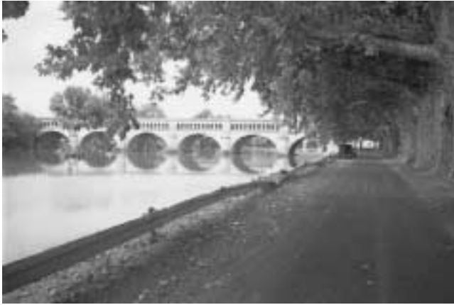
The Languedoc Canal is still in regular use 330 years after its “impossible” construction (here, one of its beautiful bridges carries the canal at Béziers near the Mediterranean terminus). Its revolutionary features included even the lining of the canal with plantain trees, whose leaves Riquet determined would provide a waterproof “cover” for the canal bottom.
