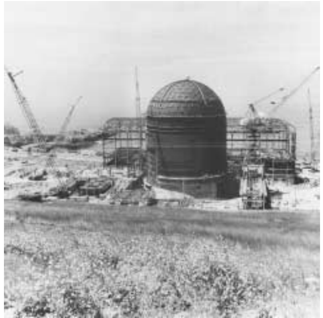
The Diablo Canyon nuclear plant, under construction by Westinghouse Electric in 1971. Built on a 750-acre complex in San Luis Obispo County, the plant’s lead-time took over 15 years, to account for seismic activity and the Pacific Ocean site. The two units are Pressurized Light Water Reactors, with a capacity of 1,087 MW each, and went on line in 1985 and 1986, respectively.
