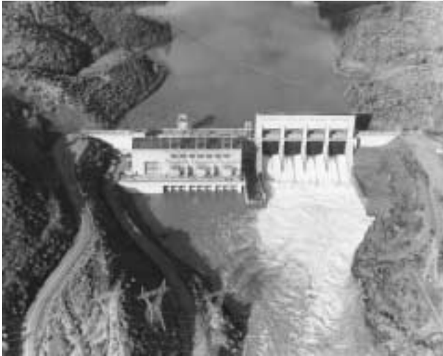
Aerial view of Keswick dam and power plant on the Sacramento River. The plant has three generating units with a total capacity of 75,000 kW (kilowatts).
