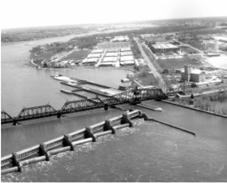
Lock and Dam 15 at Rock Island, Illinois on the Mississippi River, one of a system of 37 aging navigation infrastructures on the Upper Mississippi which need modernization with new technology, both for increased river freight traffic and to improve the ecology of the river's basin.
