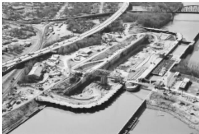
*The U.S. Army Corps of Engineers has dozens of aged locks and dams to replace and renovate on the Ohio River—if it weren't seeing its budgets cut, in absolute terms, under Bush-Cheney, and laying off instead of hiring engineers. Here's one stalled project in which the Corps is trying to replace the old and failing McAlpine Lock at the right, near Louisville, with a modern 1,200-foot lock, at left.*
