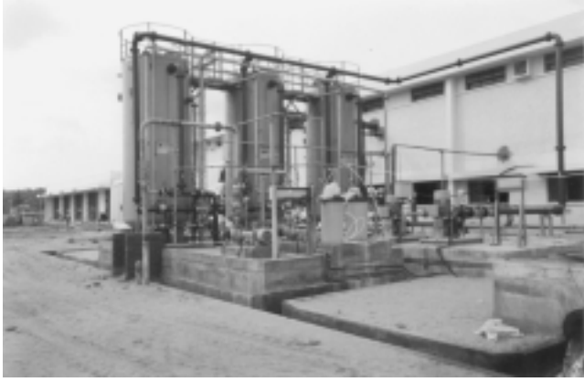
The sabotage efforts delayed, but did not stop, nuclear desalination. This 1,800 cubic meter/day nuclear-powered desalting plant is in Kalpakkam, India, a project of the Bhabha Atomic Research Center, and there are several projects on the drawing boards in other countries.
