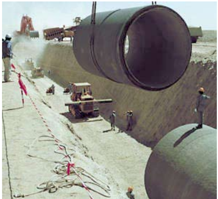
Huge, 4-meter-diameter pipes, like this one in Libya's "Great Man-Made River" project, provide a model for what can be done in Sudan, where the pipes can be much smaller (1 meter), and travel shorter distances.
