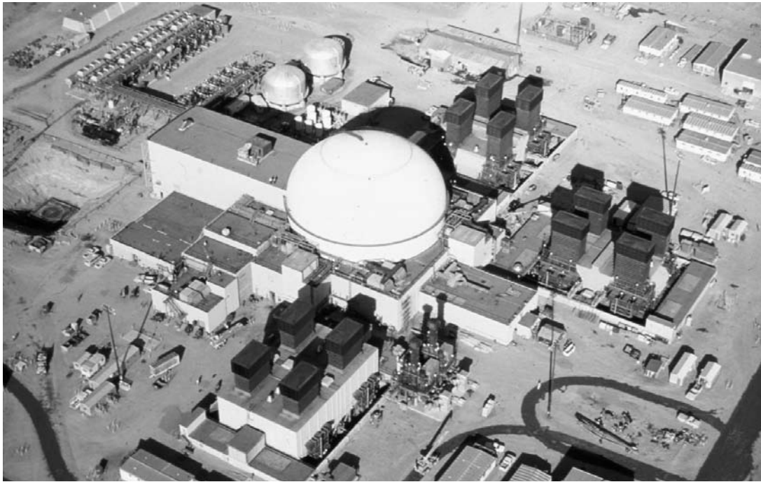
The Fast Flux Test Facility at Hanford, Washington, is a 400-megawatt sodium-cooled fast reactor of the type GNEP proposes to develop. It was designed to test new reactor fuels and materials, but it was shut down by the DOE just months before GNEP was announced. Now, it could be restarted.
