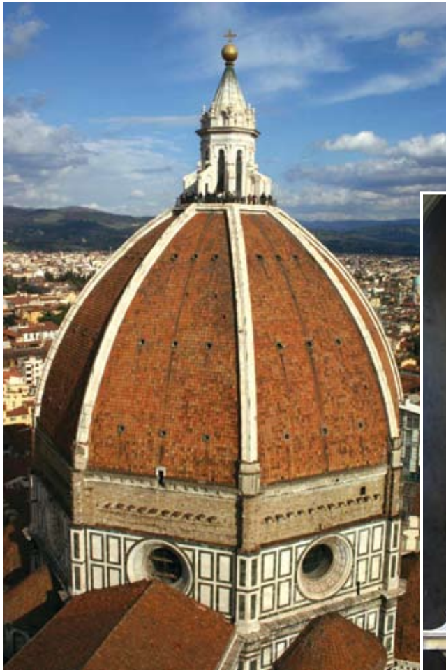
The dome on Florence's cathedral, Santa Maria del Fiore completed in the 1440s, represents a scientific breakthrough, as well as a work of beauty, constructed with the use of the catenary curve. The architect, Filippo Brunelleschi, has his own statue in the surrounding plaza, looking up at his achievement.
