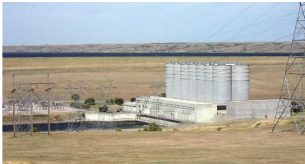
The Oahe Powerhouse, a hydroelectric plant at the Oahe Dam, near Pierre, S.D.
