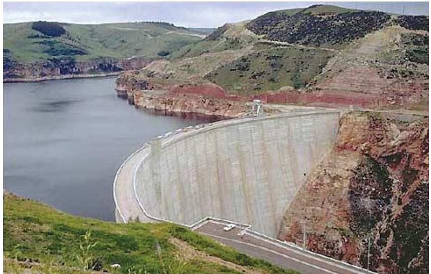
The Bureau of Reclamation’s Yellowtail Dam across Bighorn Canyon in southeastern Montana. This is the largest concrete dam in the Missouri River System.
