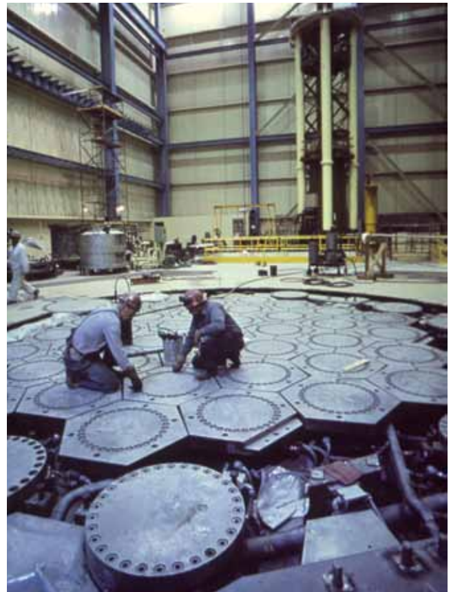
FIGURE 2 Refueling Floor, Fort Saint Vrain Nuclear Power Plant
