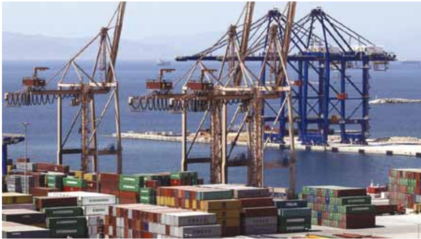
The Chinese company COSCO is upgrading Piraeus into the largest port in the Mediterranean, a gateway for East-West trade.
