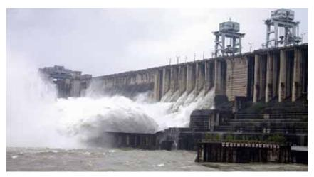
The Danjiangkou Dam on the Han River, the principal reservoir for the middle line of the South-to-North Water Diversion Project, was heightened to increase its impoundment volume, over a construction period from 2005 (shown here) to 2010. The dam was raised 14.6 m, from 162 m to 176.6 m.
