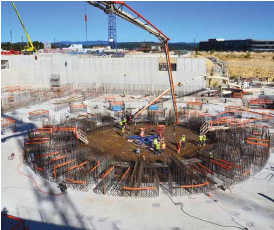
Harmony among nations: The construction of the floor of the Tokamak pit at the International Experimental Thermonuclear Reaction (ITER) site in southern France. The work is being conducted by scientists and engineers from the European Union, China, Russia, Japan, India, South Korea, and the United States.
