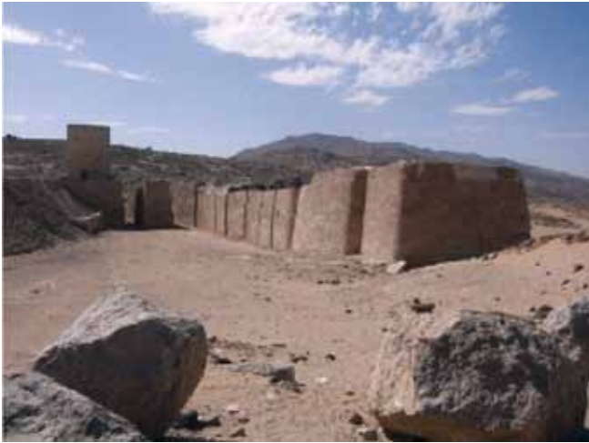
Fig. 15 The vestiges of the big dam at Marib.
