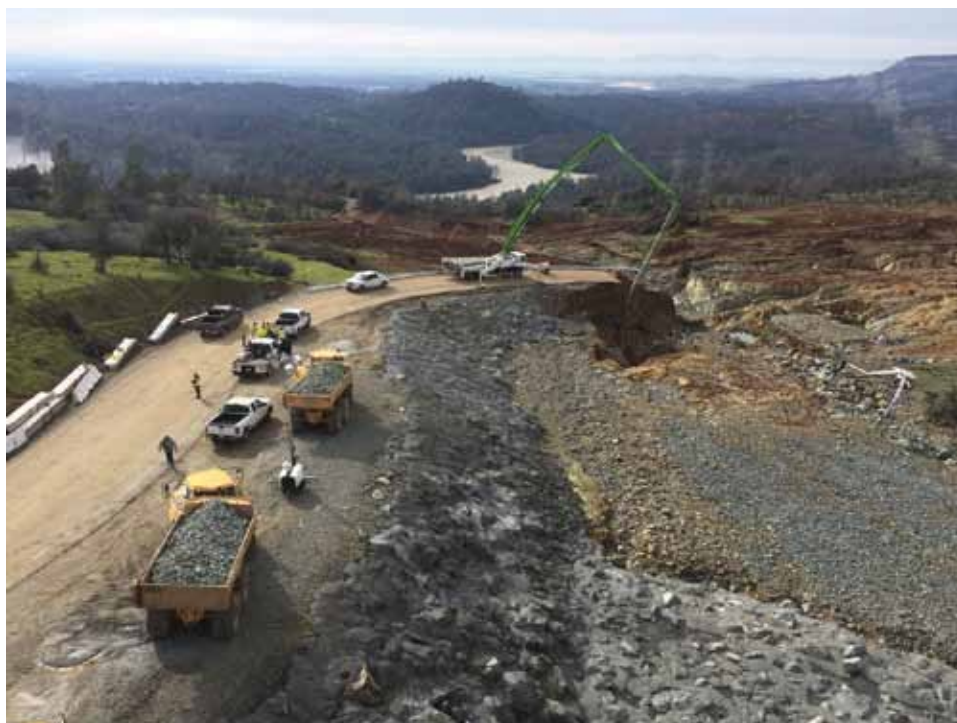
Concrete reinforcement being applied to the emergency spillway of the Oroville Dam during the crisis at the dam in 2017.
