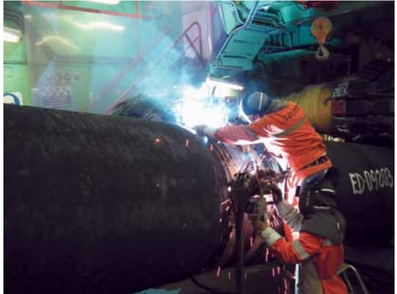
Welding pipe segments together for Nord Stream 1 on the Castoro Sei pipelaying vessel, 2011.
