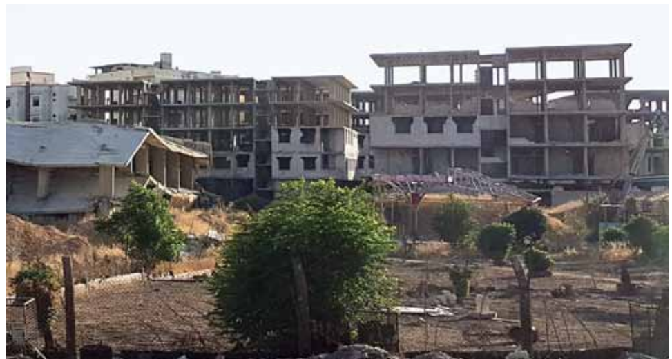
Every destroyed apartment house that could be seen in the Damascus war zones, formerly occupied by gunmen, was under repair.
