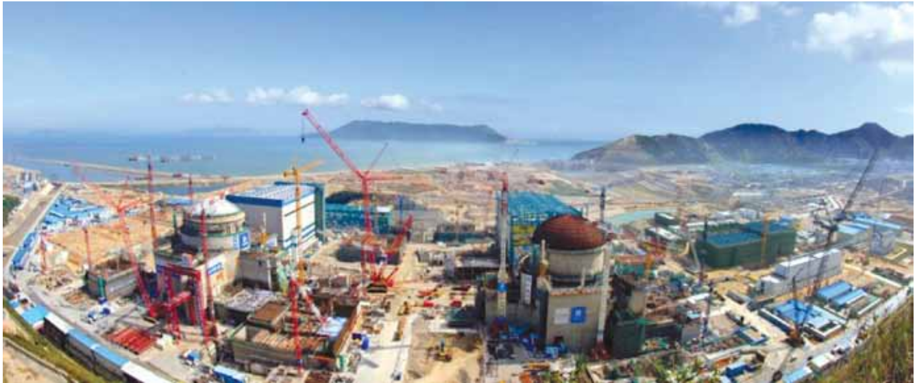
The two-unit Taishan nuclear power project, using advanced, third-generation nuclear power technology, under construction in Chixzhen, Taishan, Guangdong province, China. It is a China-foreign joint project with large participation by Areva and Electricité de France. The bulk of French electricity production is nuclear powered. France exports electricity to Germany, which is stupidly shutting down all its nuclear plants by 2022.
