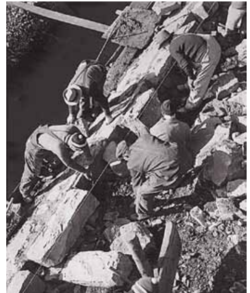
Works Progress Administration (WPA) construction.
