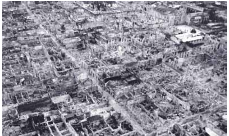
U.S. Army photo showing destruction of the Walled City district of Old Manila in May, 1945, after the Battle of Manila.
