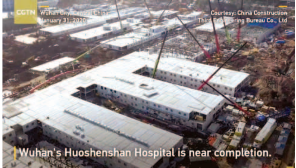
Construction of the thousand-bed Huoshenshan emergency field hospital for COVID-19 patients was begun on Jan. 23 and completed on Feb. 2, with thousands of workers working around the clock. This photo was taken on Jan 31. Leishenshan Hospital, built with the same design, was finished on Feb. 8.
