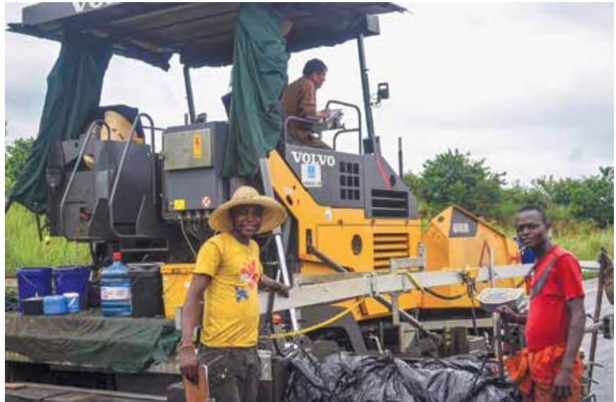
The Republic of the Congo’s No. 1 National Highway, constructed by the China State Construction Engineering Corporation and completed March 1, 2016, connects the deep-water port of Pointe-Noire to the inland capital city, Brazzaville. Here, an asphalt paver at work on a section of that road.
