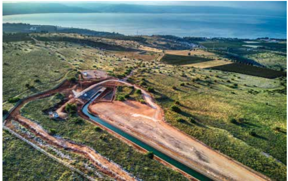
The Hukok Canal portion of Israel's National Water Carrier transfers 72,000 cubic meters per hour of fresh water from the Sea of Galilee in the north to the highly populated center and the arid south. April 28, 2023.
