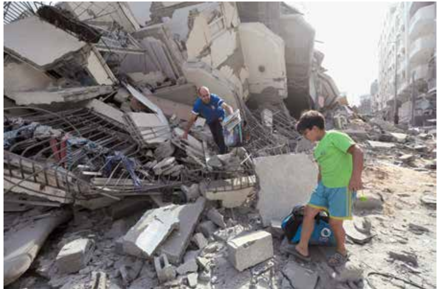
Wafa Palestinians inspect the ruins of the former ten-story, residential Al-Aklouk Tower, destroyed in Israeli Air Force strikes. Gaza City, Oct. 8, 2023.
