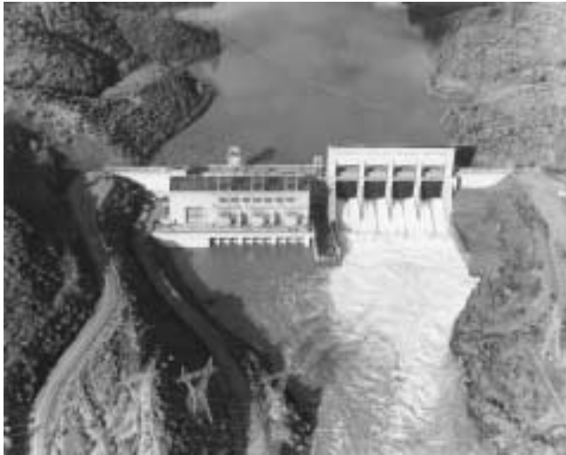
Aerial view of Keswick dam and power plant on the Sacramento River. The plant has three generating units with a total capacity of 75,000 kW (kilowatts).
