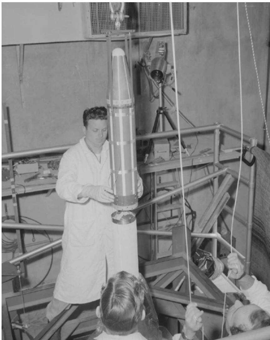
The Explorer-1 satellite, seen here being lowered onto the rocket's fourth stage, in preparation for launch, housed a 30-pound science payload. Dr. James Van Allen's on-board Geiger counter made the first scientific discovery of the Space Age—bands of radiation belts around the Earth.
